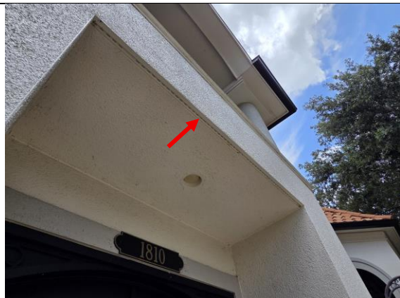
NOTE: The front entry soffit has drainage provision.
