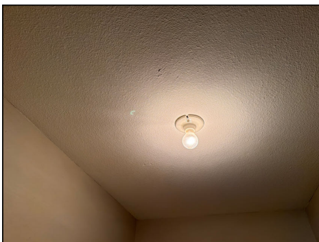
Current standards require globes on closet fixtures
