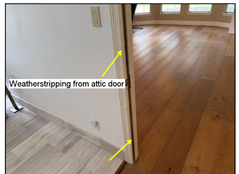
Upstairs right rear area appeared to be converted attic space
