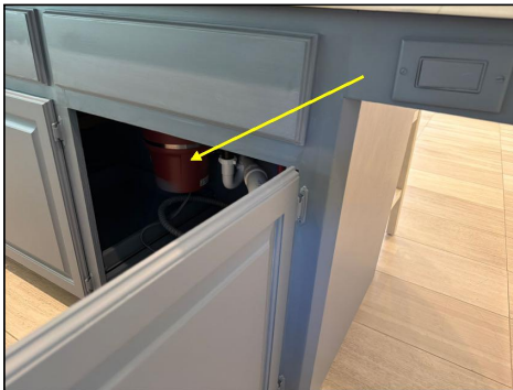
Disposal switch noted to be right of the island sink
