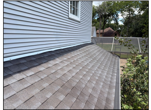
Roofing materials appeared to be performing as intended
