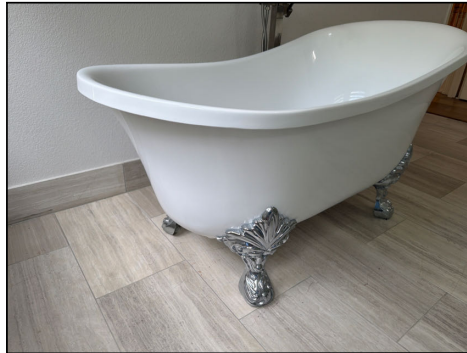
Upstairs right tub is loose at the floor/Easily moves
