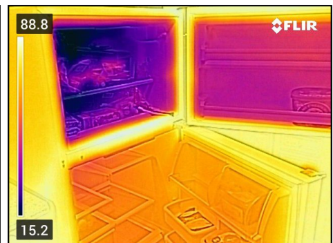
The refrigerator/freezer appears to be operative
