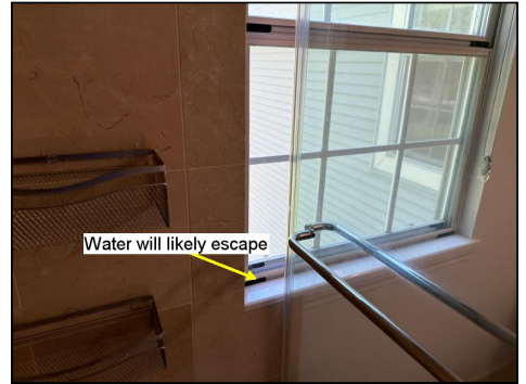
Less than ideal configuration at the left secondary shower surround
