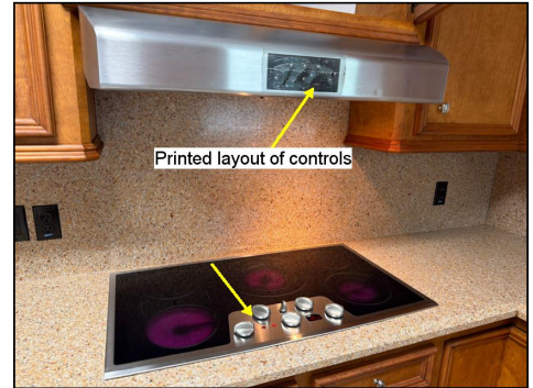
Controls faded at garage cooktop
