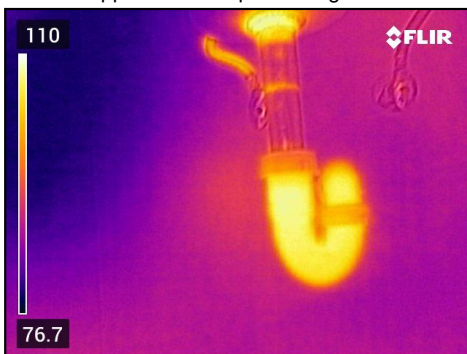
Drains appeared to be performing as intended
