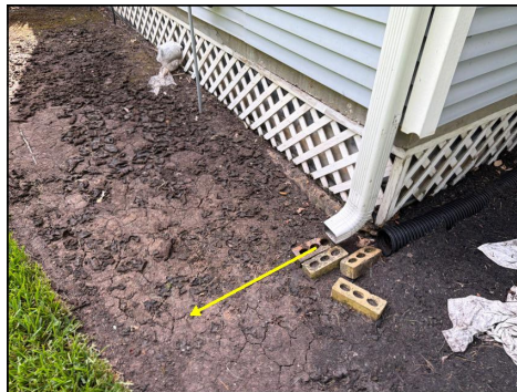
Gutter extensions are recommended
