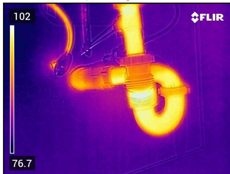
Drains appeared to be performing as intended
