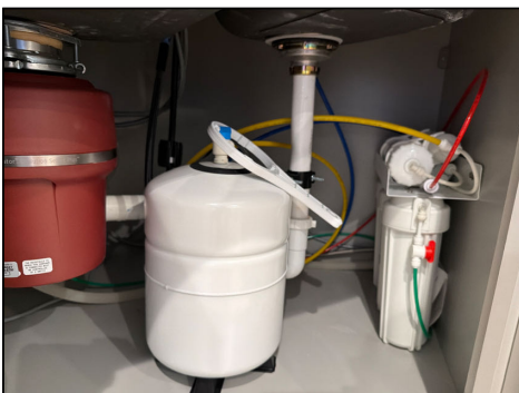
Water filtration system was not inspected
