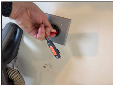
Rear garage dryer outlet appeared to be performing as intended
