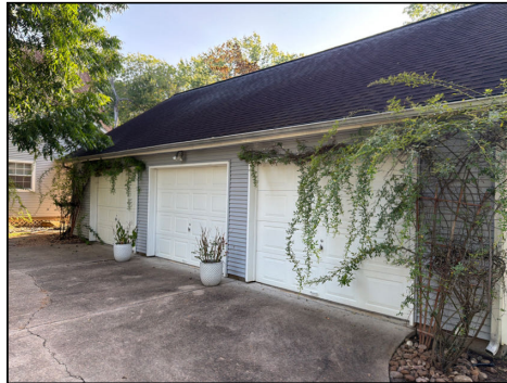
Foliage is recommended to be cut back and kept clear of the exterior walls
