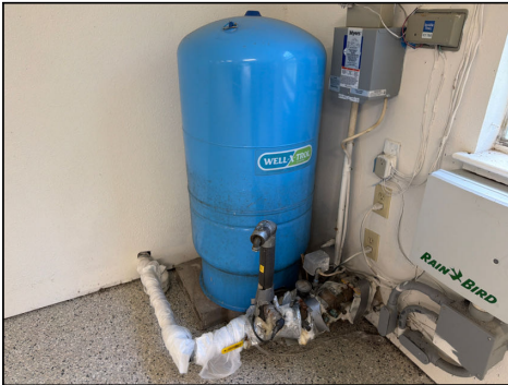
Well should be further evaluated for low pressure
