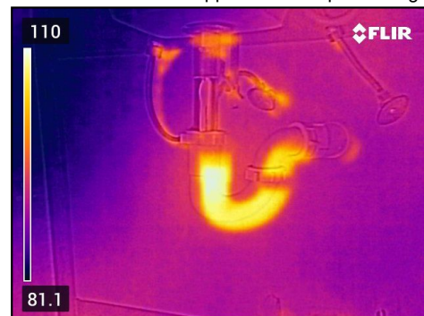
Drains appeared to be performing as intended
