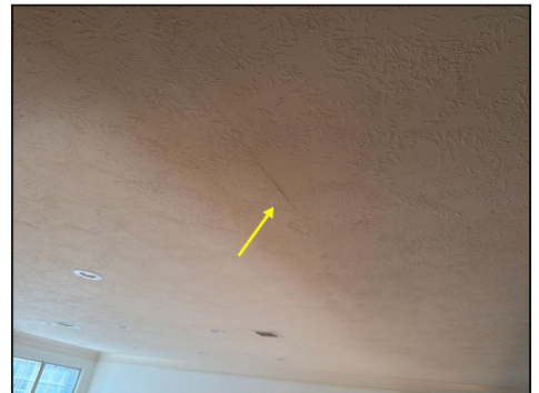
Damaged drywall/cracked seam observed at the family room ceiling
