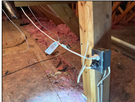
Extension cord used as permanent wiring in the attic
