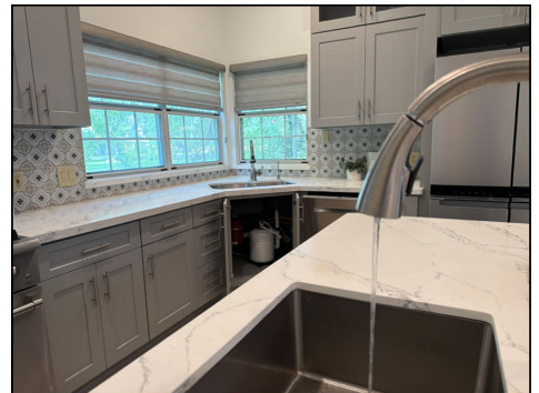
Low water pressure noted at the fixtures throughout the home
