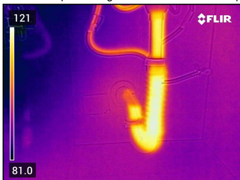
Drains appeared to be performing as intended
